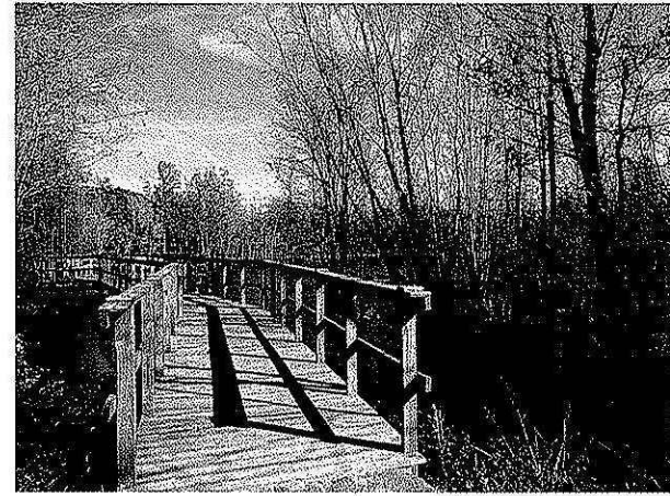
Lorain County Metro Park
